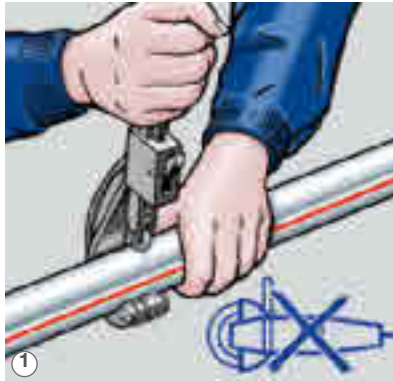
① Stripped Prestabo-pipe cut the pipe to length at as near to a right angle as possible
