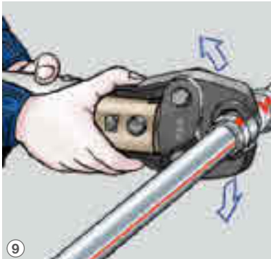
Once press connection complete, open the press jaw.
